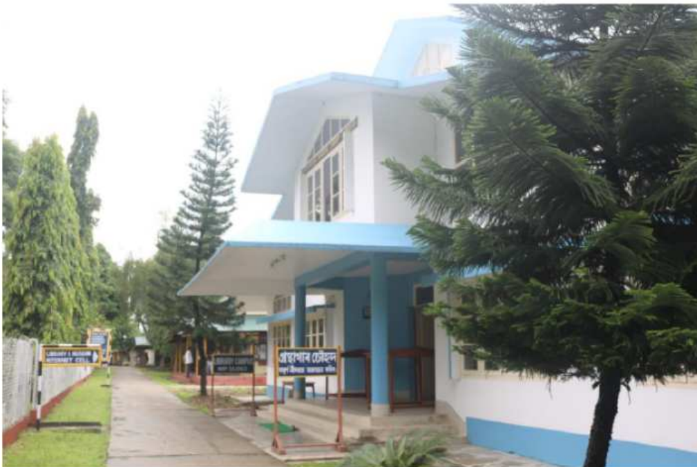
Front View of the Library
